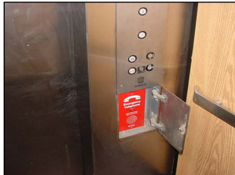
Elevator emergency phone with compartment.
